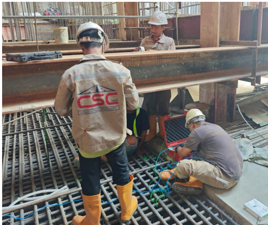
Figure 40: Monitoring Station, Sensor Installation
