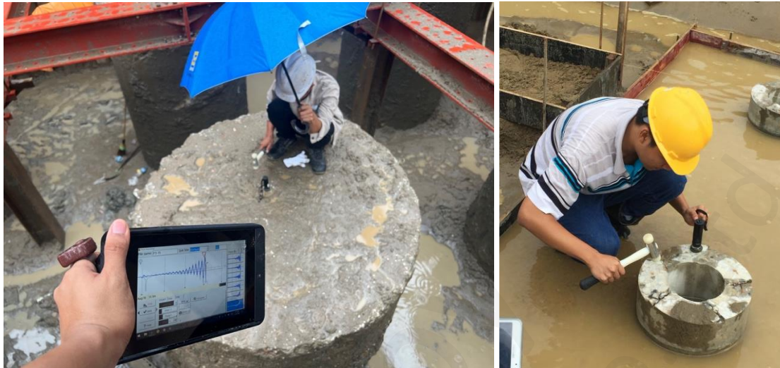
Figure 3: PIT Testing on Bored Pile (Cast in-situ Piles), Pre-casted Piles
