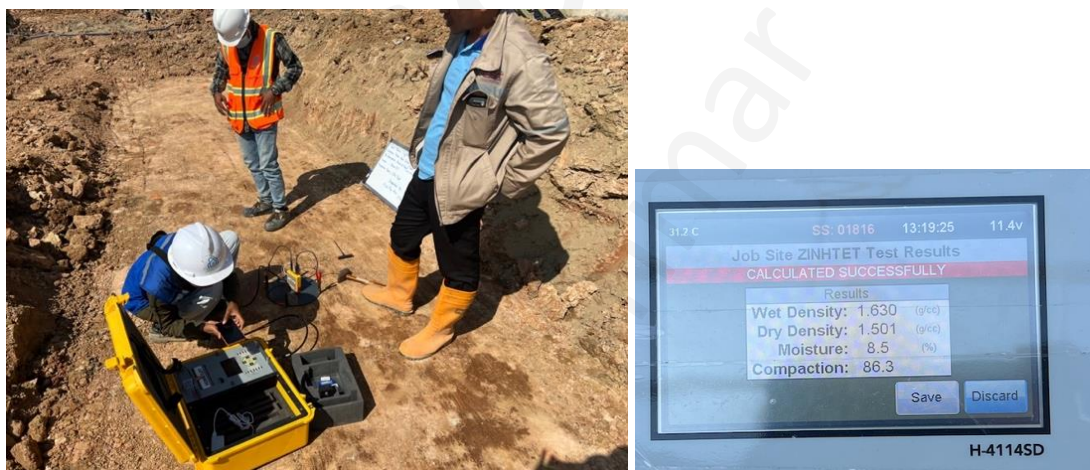
Figure 23: Performing Soil EDG Tests
