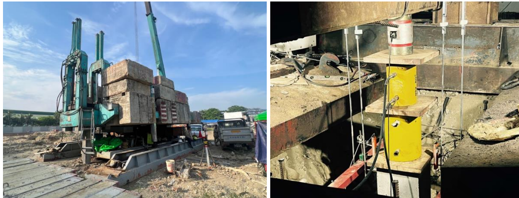
Figure 19: Piling Machine as a Kentledge Counterweight
