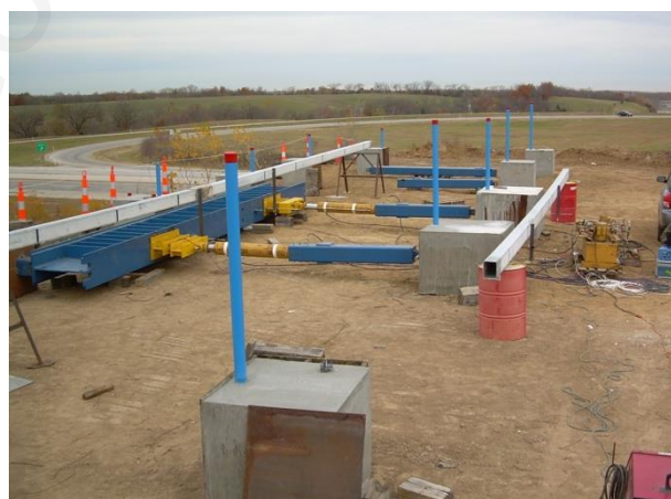
Figure 21: Pile Static Lateral Load test
