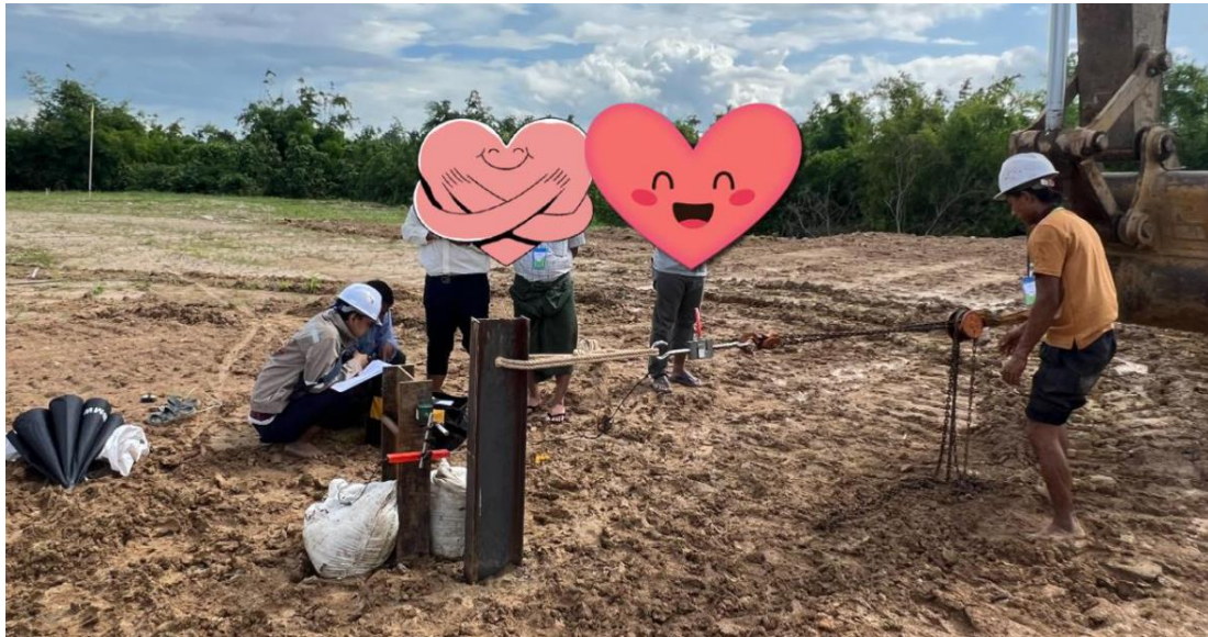
Figure 34: Solar Foundation Pull Out & Lateral Test
