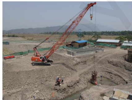
Pile Dynamic Load Test
