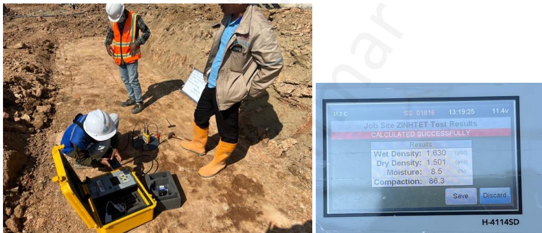
Figure 23: Performing Soil EDG Tests
