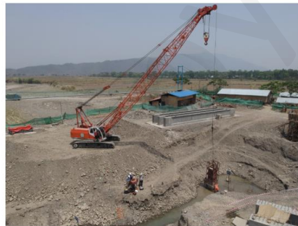
Pile Dynamic Load Test
