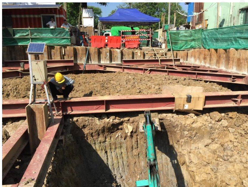
Figure 33: Struct Force Monitoring Station @ Deep Excavation Site
