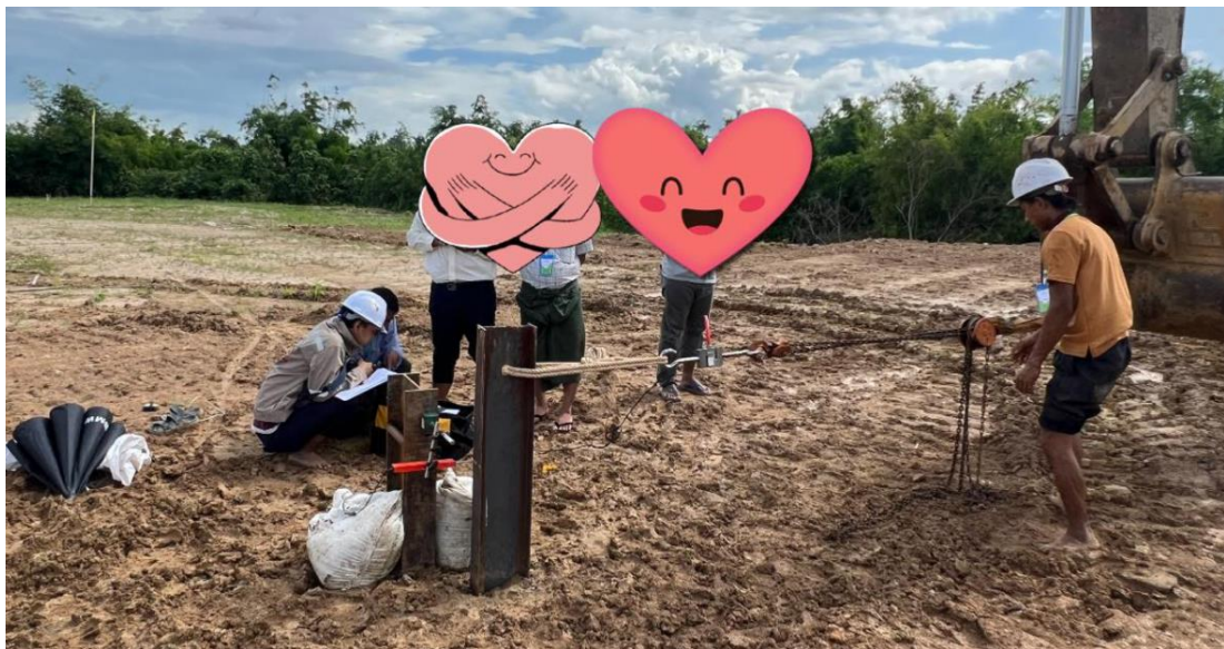
Figure 34: Solar Foundation Pull Out & Lateral Test
