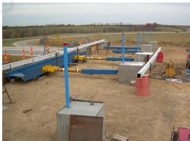
Figure 21: Pile Static Lateral Load test
