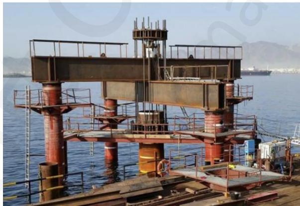
Figure 20: Pile Static Axial Tension Load test
