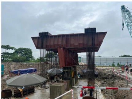
Pile Static Load Test
