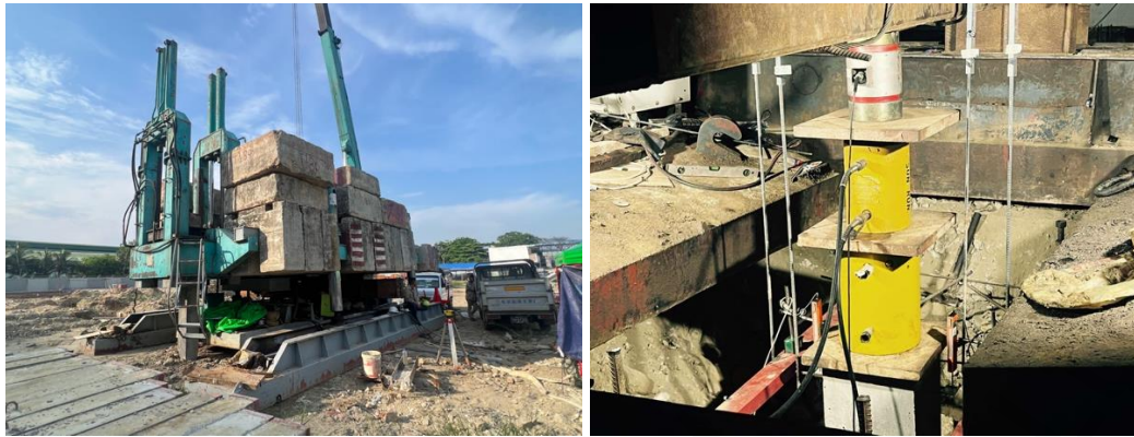
Figure 19: Piling Machine as a Kentledge Counterweight
