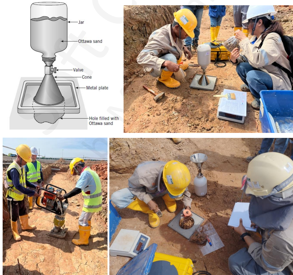
Figure 83: Sand Cone Test Equipment & Testing Photos
