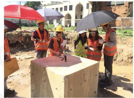
Pile Integrity Test
