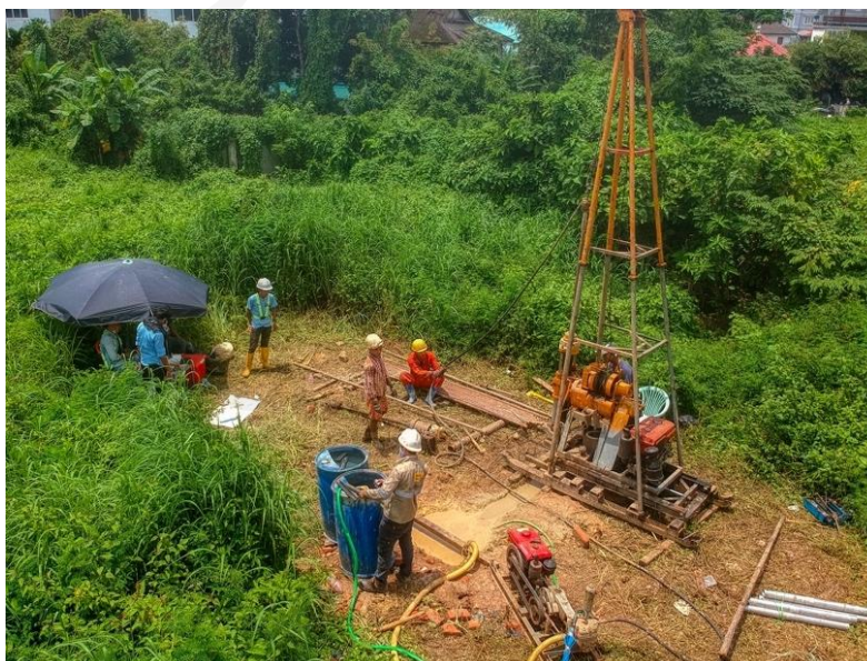
Figure 60: Rotary Wash Boring Setup for Deep Boring
